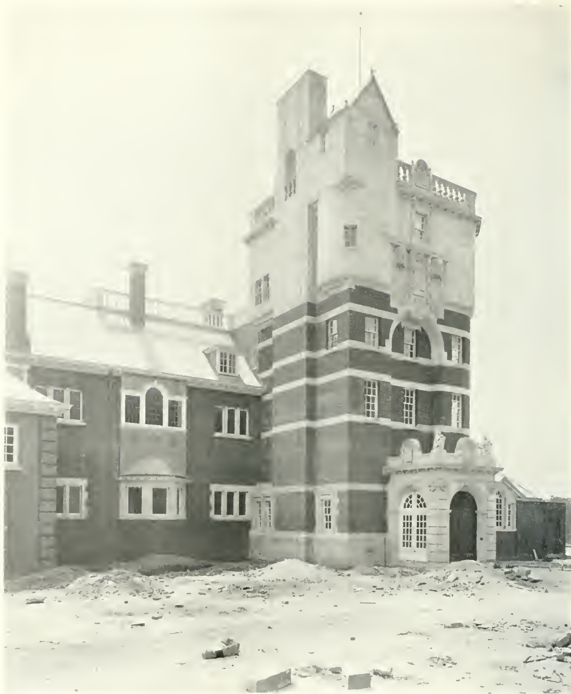
THE TOWER PANGBOURNE VIEW OF THE NORTH ENTRANCE.
